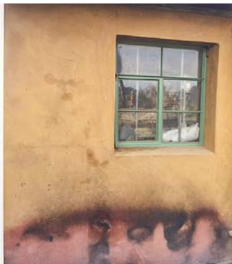
Clockwise from top left: Norrbon Road straw bale home (Photo: Edward Caldwell/Arkin Tilt Architects). Fires burned to the footings but not up the walls. The mineral oxides in natural hydraulic lime turn pink when heated, showing where the fire reached. (Photos: Michel Courveaux/TransMineral). Straw bale home on Lovall Valley Loop Road withstood fire against its walls. Photos courtesy of CASBA – The California Straw Building Association.
