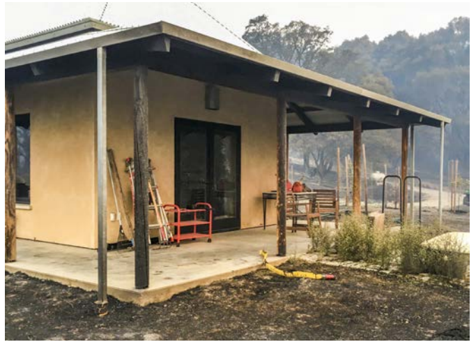
Redwood Valley residence – columns salvaged from a prior fire frame the conflagration, they charred but did not ignite. (Photos: Edward Doody/Arkin Tilt Architects. Courtesy of CASBA – The California Straw Building Association)
