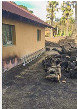
Clockwise from top left: Norrbon Road straw bale home (Photo: Edward Caldwell/Arkin Tilt Architects). Fires burned to the footings but not up the walls. The mineral oxides in natural hydraulic lime turn pink when heated, showing where the fire reached. (Photos: Michel Courveaux/TransMineral). Straw bale home on Lovall Valley Loop Road withstood fire against its walls. Photos courtesy of CASBA – The California Straw Building Association.
