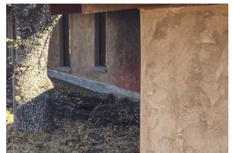
Clockwise from top left: Norrbon Road straw bale home (Photo: Edward Caldwell/Arkin Tilt Architects). Fires burned to the footings but not up the walls. The mineral oxides in natural hydraulic lime turn pink when heated, showing where the fire reached. (Photos: Michel Courveaux/TransMineral). Straw bale home on Lovall Valley Loop Road withstood fire against its walls. Photos courtesy of CASBA – The California Straw Building Association.
